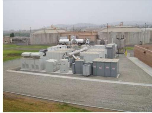
power plant was an important aspect of their purchasing decision. The efficiency of fuel cells can exceed 80% when by-product heat is utilized and, due to the lack of combustion, virtually no harmful NOx, SOx or particulate matter pollutants are emitted by the fuel cells.
